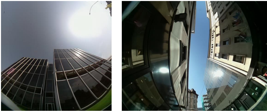
Figure 3 & 4 Solar reflection on glazed facades in an open area (figure 3) and in a narrow canyon (figure 4)
